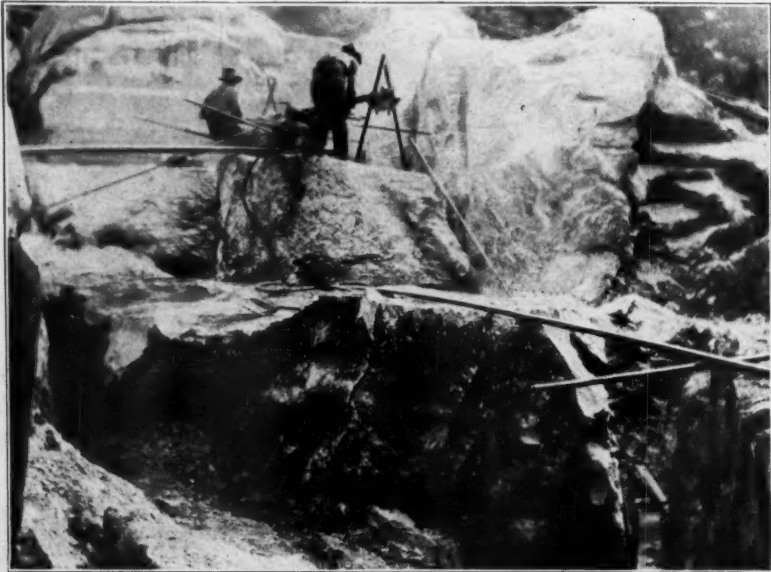
Drilling In on Solid Ledge of Marble
